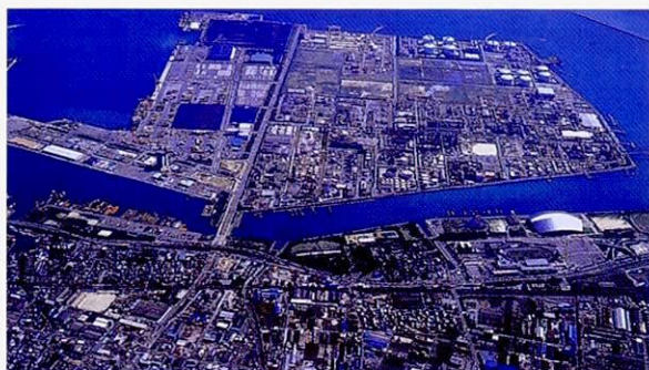
Kasumi Industrial Complex
