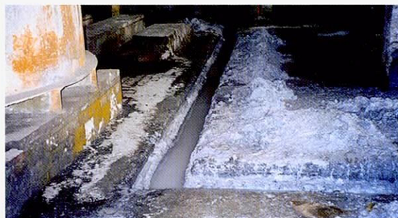
Wastewater drainage in the fertilizer factory
