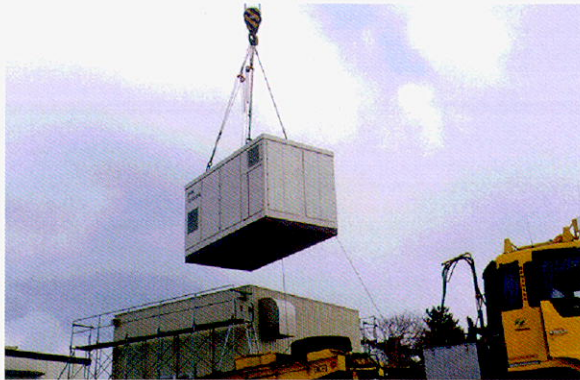
Photo 1: LPG fueled fuel cell power plant
